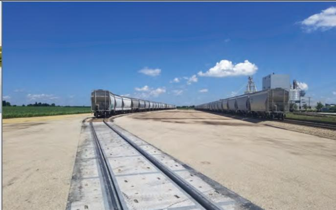
The Rochelle Transload Center (RTC) is a rail-truck transload site that can accommodate 60 cars on two tracks. This site is capable of handling shipments including dry bulk, liquid bulk, dimensional, oversized, machinery, metals and other commodities and products.
